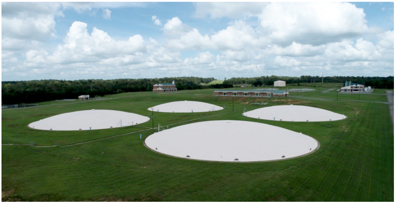
Each of the four clear wells at Frank C. Amerson, Jr. Water Treatment Plant hold 5 million gallons of finished water.
