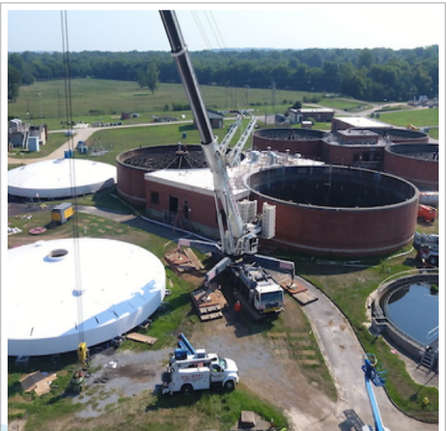
Digester lid replacement, Lower Poplar Reclamation Plant
